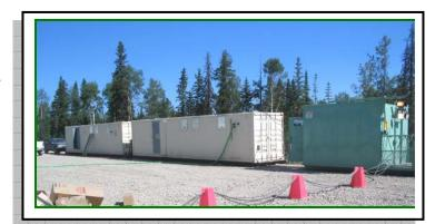
The 50-person wastewater treatment technology is housed inside a standard 40' ISO shipping container and based on this core model numerous sizing combinations are possible --- up to 500 person occupancy.
